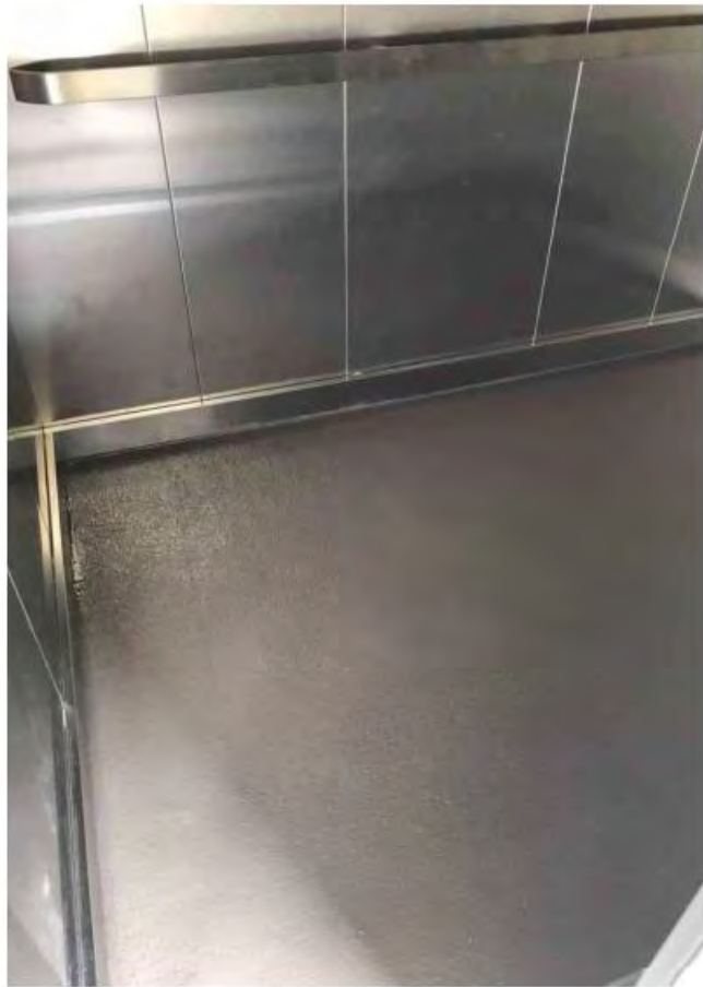
FINISH ELEVATOR FLOOR
