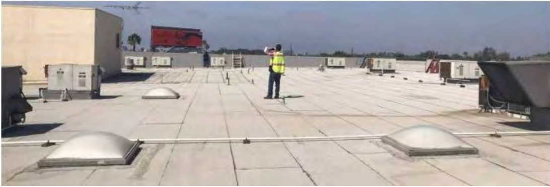
SURVEY ROOF DRAINAGE AT 6750 FOR NEW DRAINS
