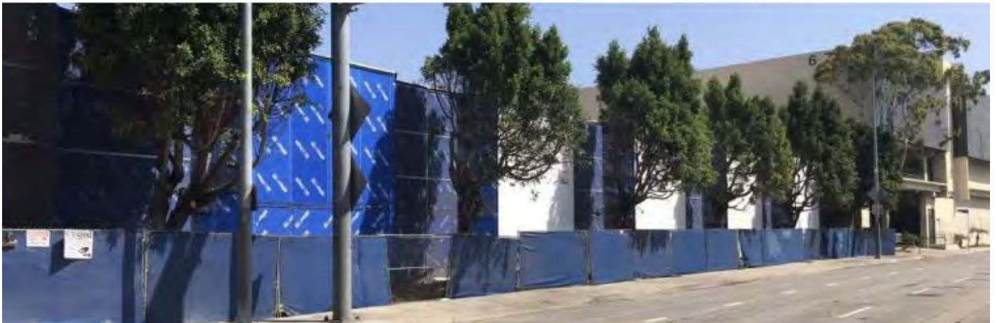
BEGIN INSTALLATION OF MOSQUITO PANELS (4 OF 10)
