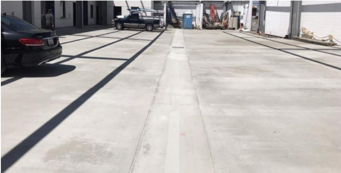
FINISH SITE DRAINAGE AND CONCRETE PLACEMENT.
