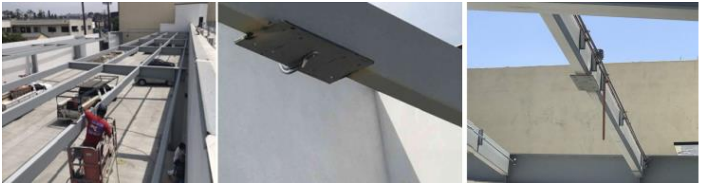
INSTALL HOSE REEL BACKING PLATES
