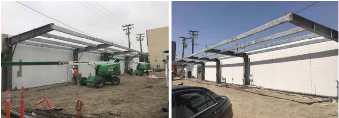
FINISH NORTH PARKING CANOPY STRUCTURE
