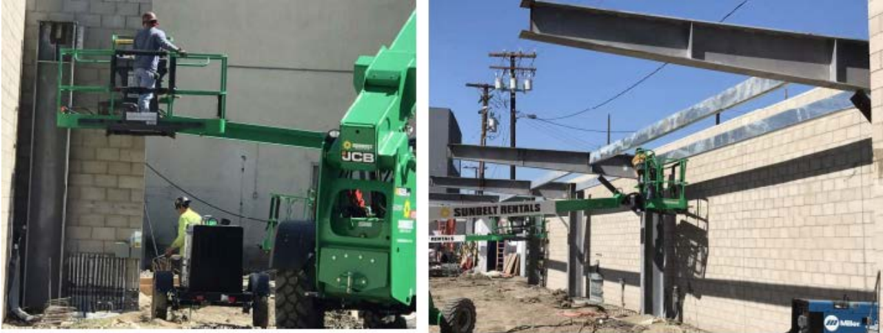
NORTH PARKING CANOPY STEEL FRAME
