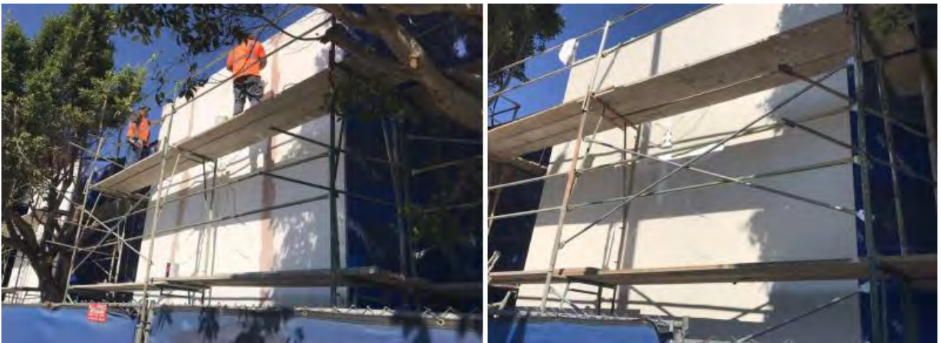
PATCH AND PAINT MOSQUITO PANELS-6740
