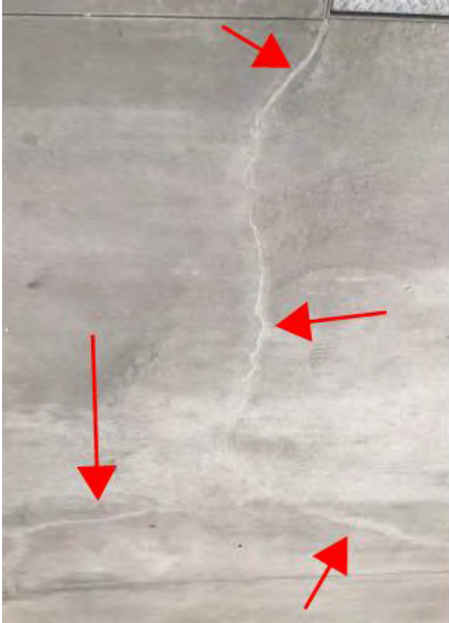
DRIVE WAY CRACKS SAMPLE REPAIRS-REJECTED
