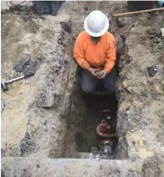
CONNECT FIRE SPRINKLER RISER TO FIRE WATER SUPPLY LINE IN THE ALLEY.
