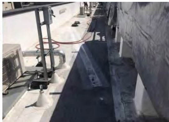
INSTALL WATER SHIELD PAN ABOVE MAIN ELECTRICAL PANEL
