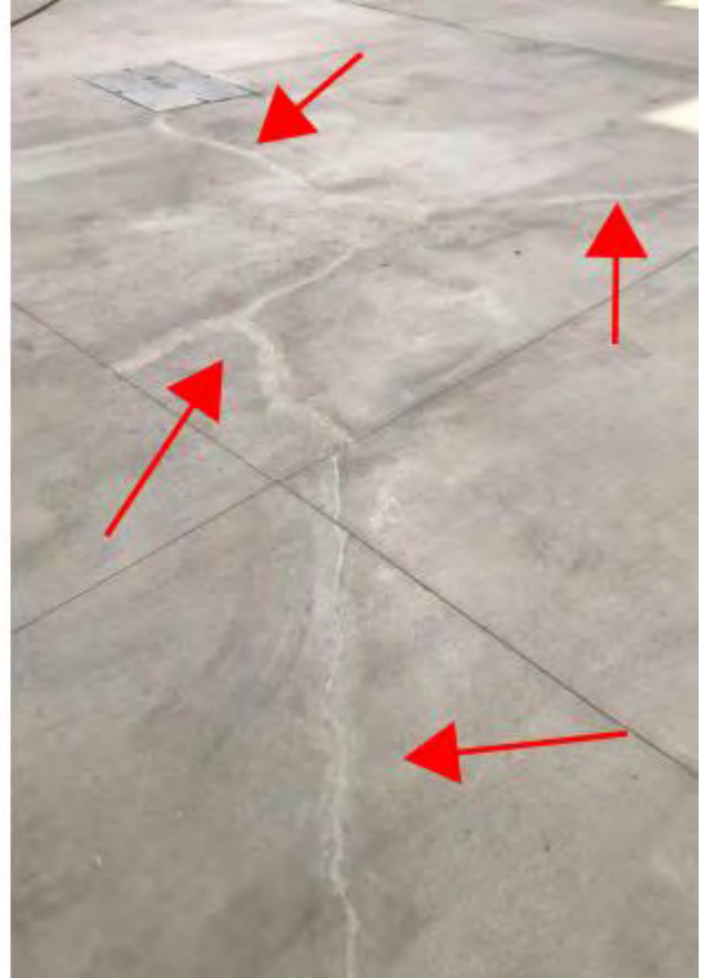
DRIVE WAY CRACKS SAMPLE REPAIRS-REJECTED
