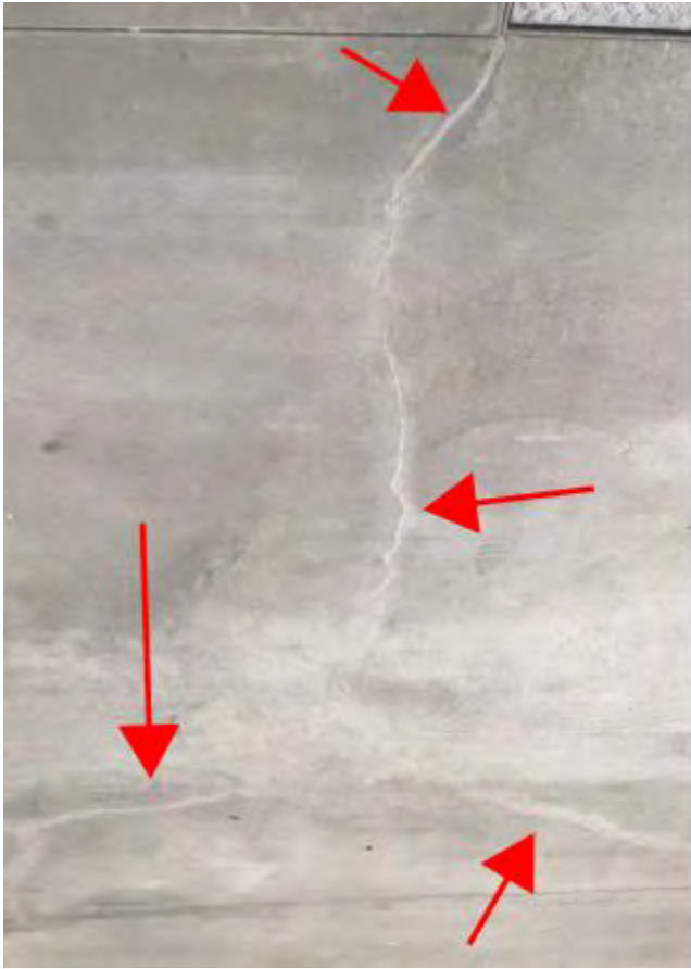
2) Drive Way Concrete Cracks
