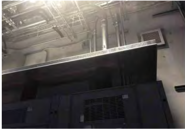
INSTALL WATER SHIELD PAN ABOVE MAIN ELECTRICAL PANEL
