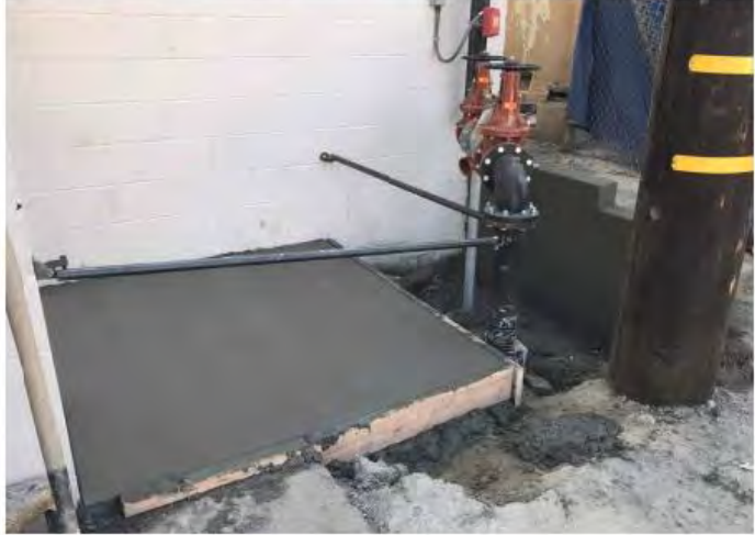
FINISH WATER CONNECTION TO FIRE SPRINKLER RISER
