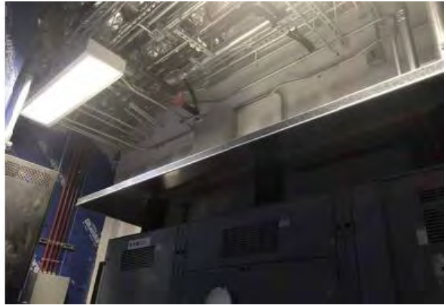
INSTALL WATER SHIELD PAN ABOVE MAIN ELECTRICAL PANEL
