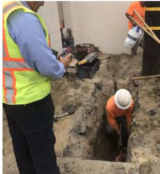
CONNECT FIRE SPRINKLER RISER TO FIRE WATER SUPPLY LINE IN THE ALLEY.
